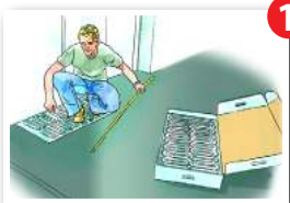
Lay out Reflect Plates
