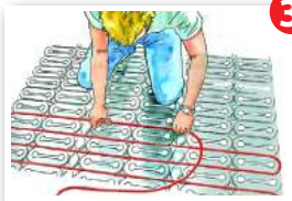
Install heating cable in grooves, pressing gently
